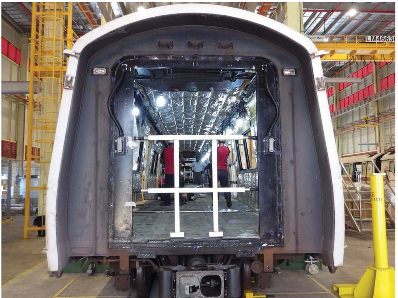
SRE engineers assess the condition of a C651 car at the Bishan depot in Singapore. The first refurbished set will be completed in early 2017.
