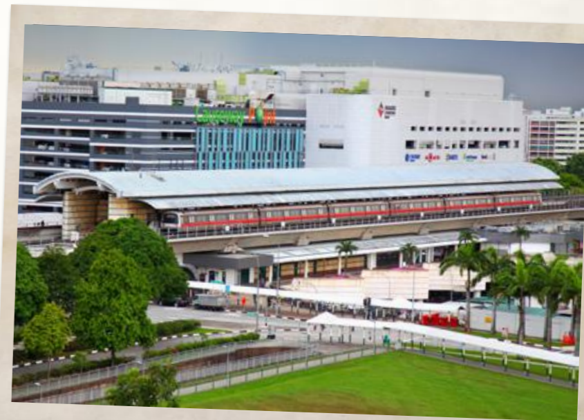
Woodlands MRT station is the only station on the Woodlands Extension with a barrel roof
