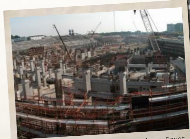
Construction of Kim Chuan Depot, home to CCL operations
