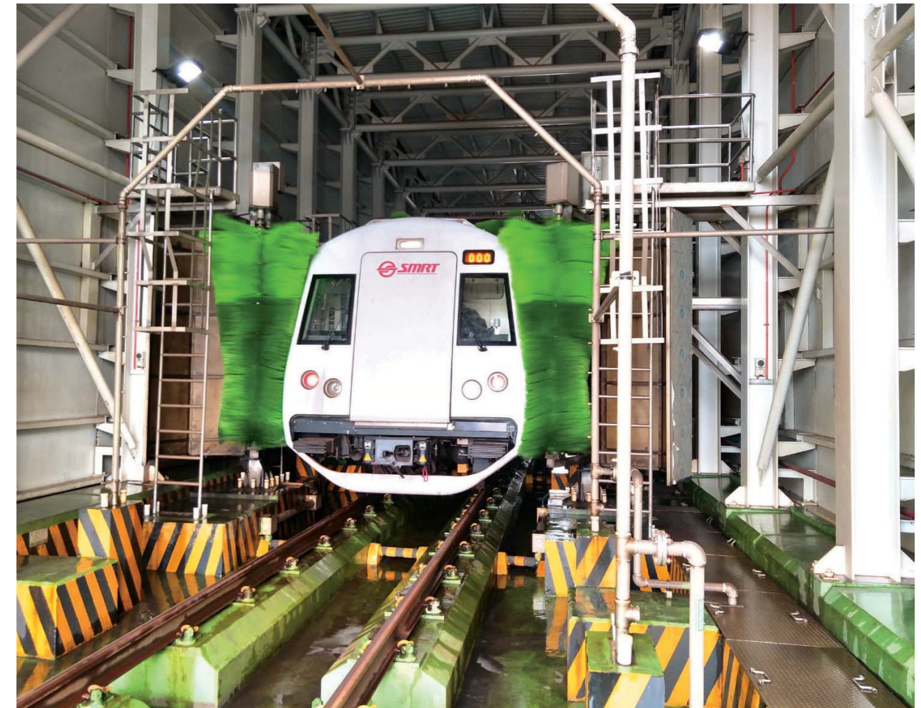
A train being washed at Bishan Depot's wash plant.
