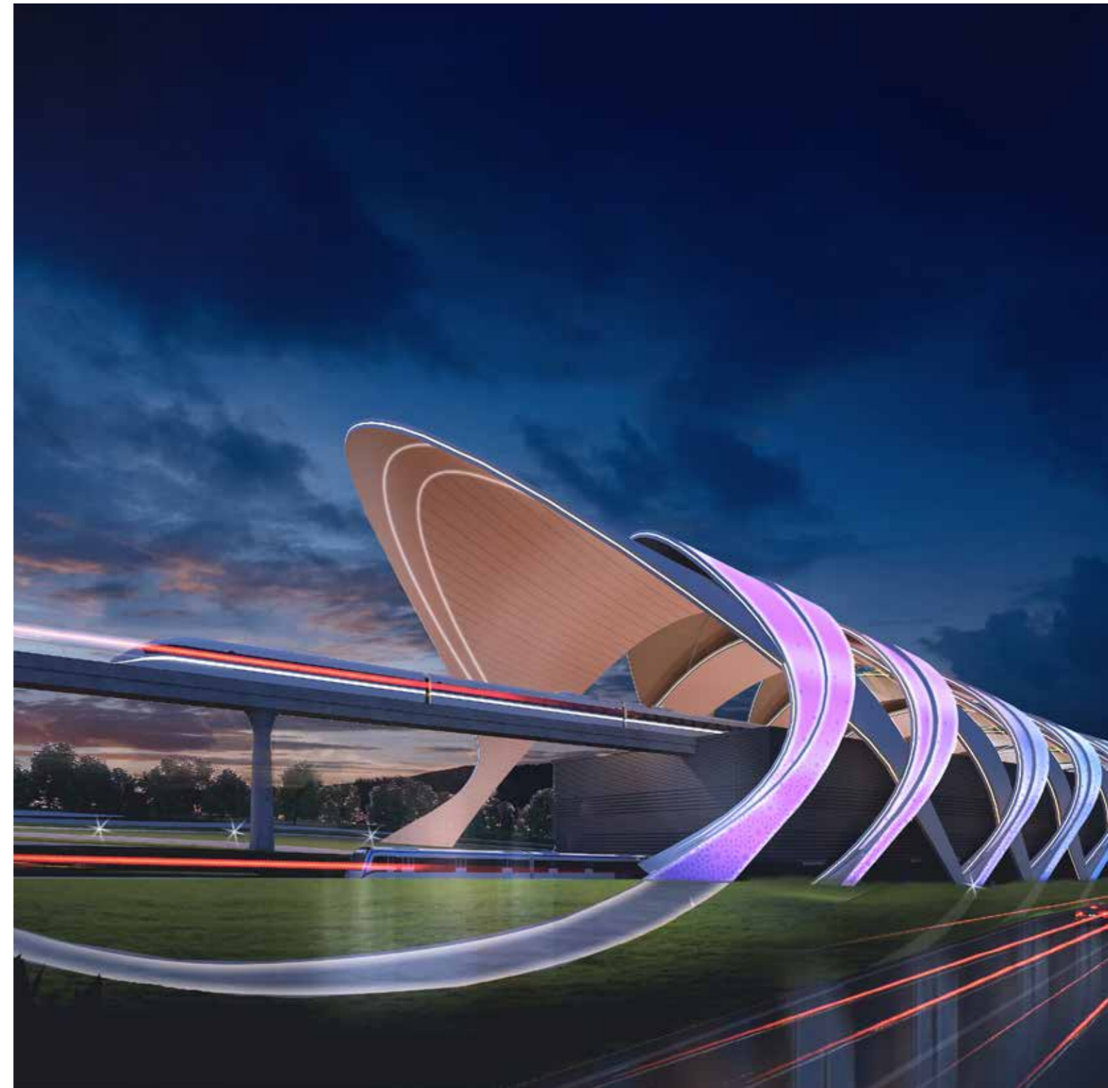
The future Johor Bahru-Singapore RTS Link Station in Bukit Chagar
