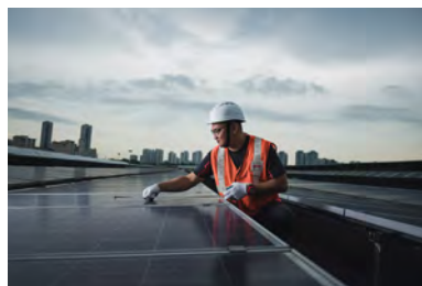
SMRT harnesses solar energy across Bishan Depot, Tuas West Depot, Mandai Depot and our TEL stations.
