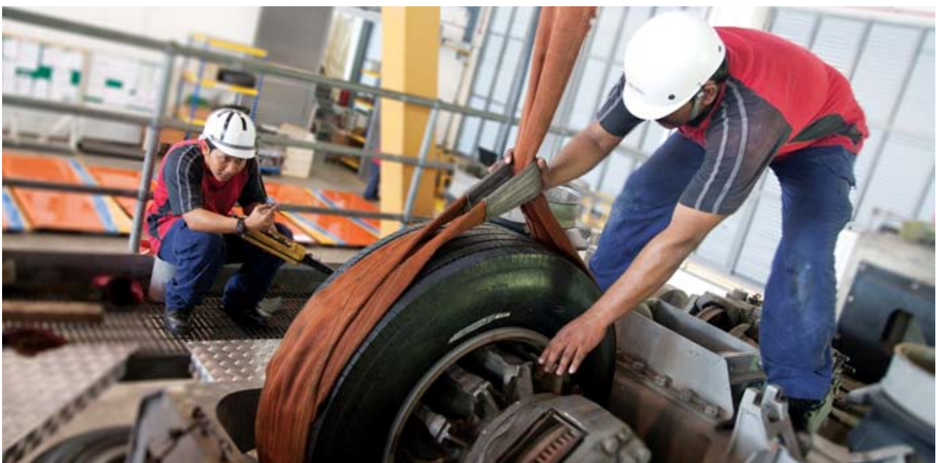
Hoisting the wheel into the bogie of the monorail
