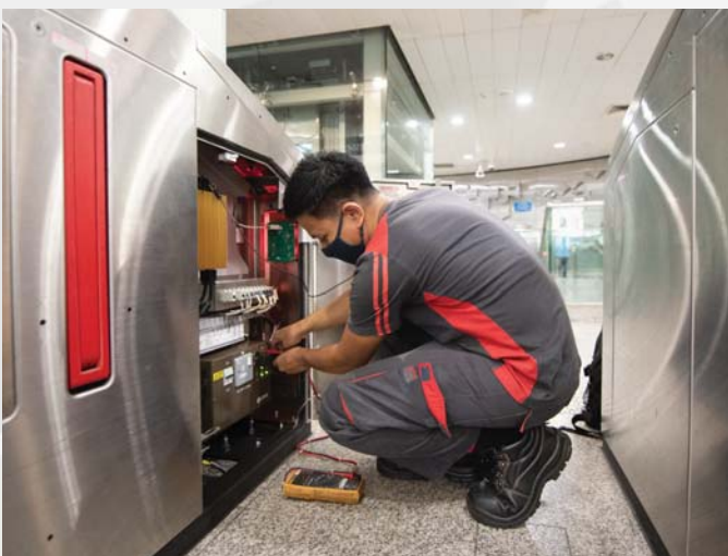
Fare System Maintenance staff performing preventive maintenance on the fare gate.
