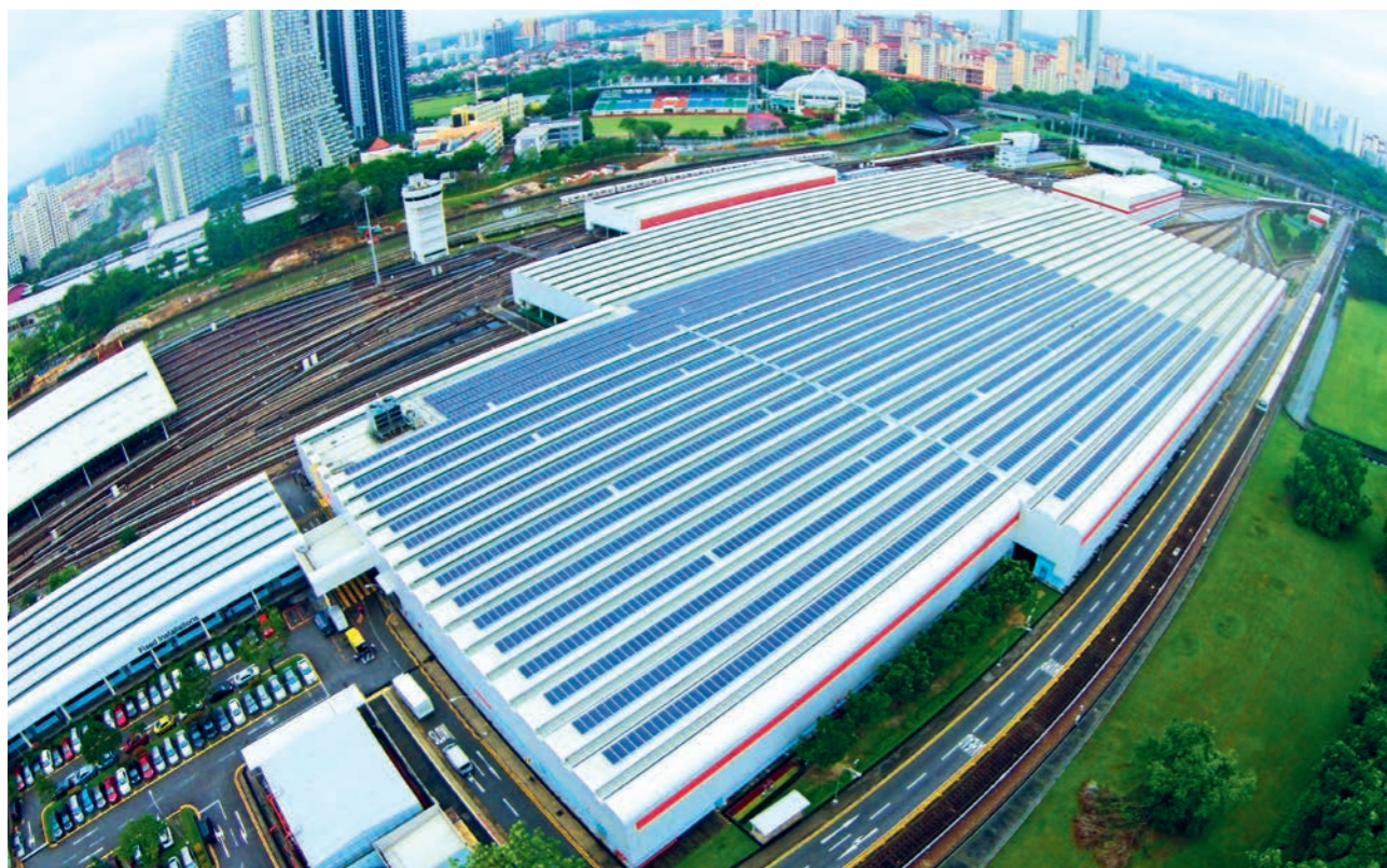
Solar PV panels in Bishan Depot: The installation of a 1MWp solar photovoltaic system covering 10,000 sq m on the main building of SMRT's Bishan Depot was completed in October 2016. It allows the depot to meet energy needs such as lighting and air-conditioning for its buildings and workshops. Photo credit: Sunseap
