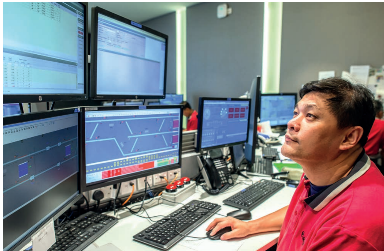
The Maintenance Operations Centre: The MOC makes use of condition monitoring tools and real-time data analytics to allow us to respond to faults more effectively.
