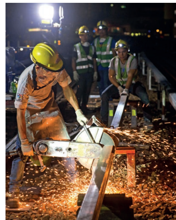
The SMRT Trains' team works through the night to replace the Power Rail.
